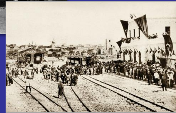
Inauguration of Jerusalem Rail Station, 1892
